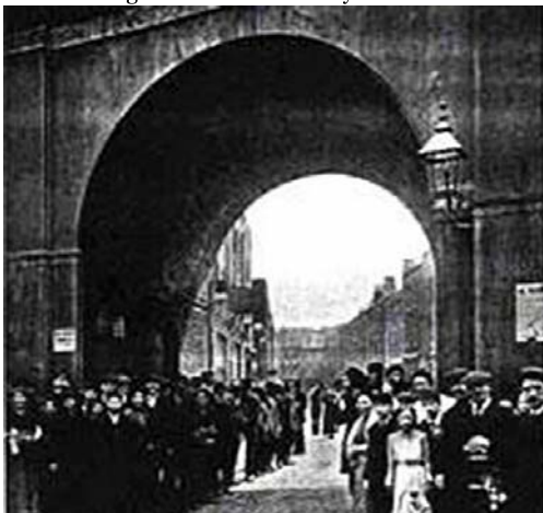
Above: The Tenter Street arch.
